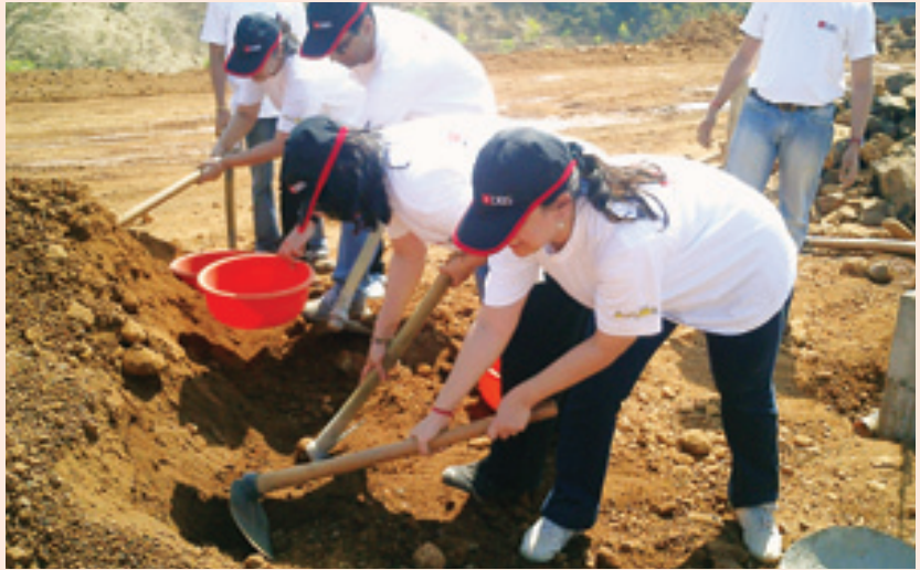
DBS staff lending a hand with the construction of an educational centre in India.
